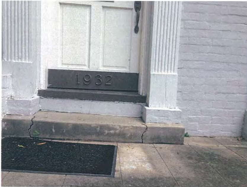
Photo3. Unleveled house foundation with cracks at main entrance. 1.5 inches drop from column to column along concrete step.
