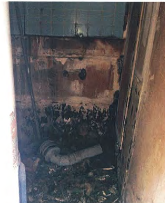
Photo18. Deteriorated walls and mold at garage apartment.
