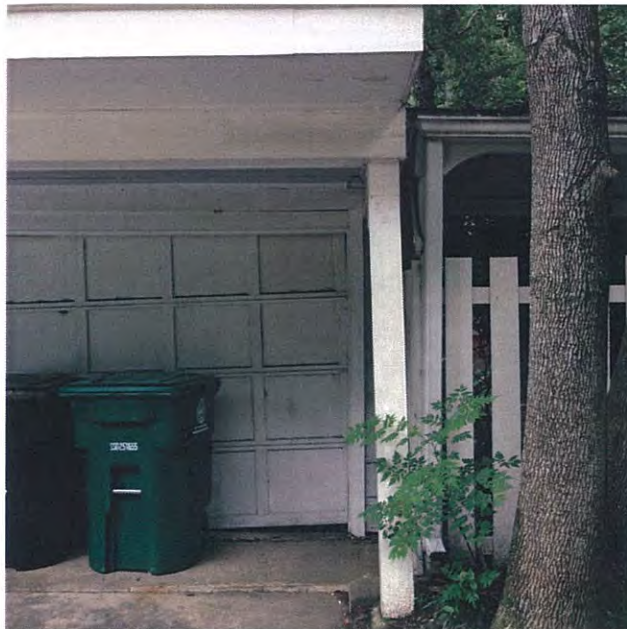
Photo16. Out of plumb column and damaged concrete slab at garage apartment
