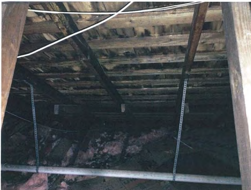
Photo12. Sagging roof framing members and moisture infiltration thru roof deck.
