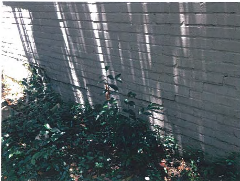
Photo4. Brick veneer crack along perimeter grade beam at main residence.
