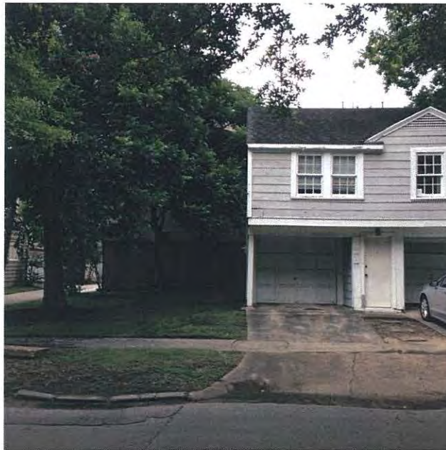
Photo17. Out of plumb column, sagging overhang and unleveled windows at garage apartment .
