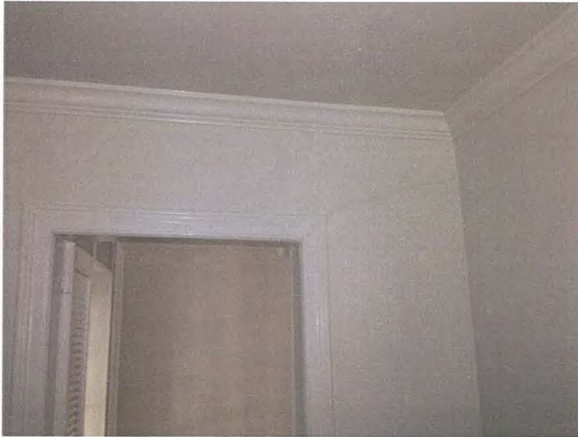
Photo9. Typical cracks at headers on doors and windows at main house
