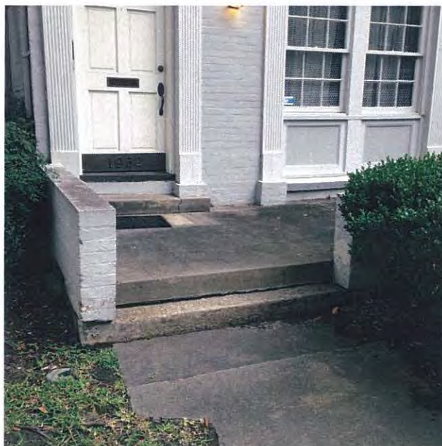
Photo2. House foundation unlevelled with cracks.
