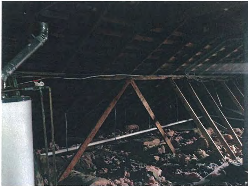
Photo13. Inadequate roof framing and bracing
