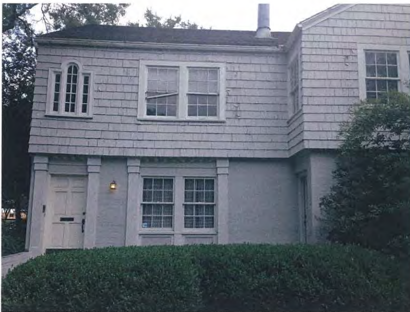
Photo1. Exterior elevation at main house on South Boulevard. Siding paint and windows are deteriorated. Second floor wall cambers down at center, windows and entrance door are unlevelled.
