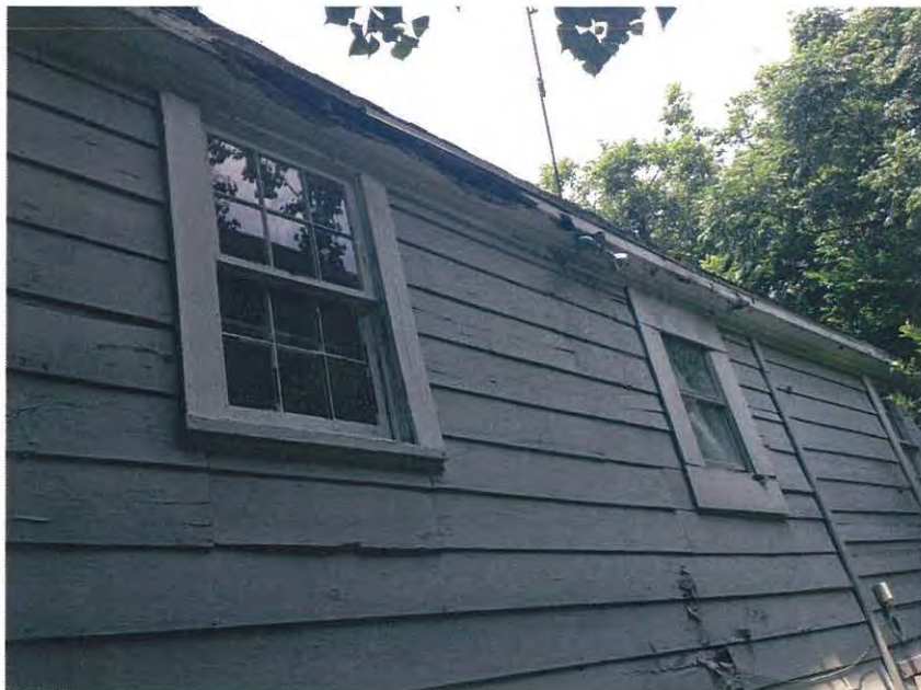
Photo14. Damaged wood siding at garage apartment.
