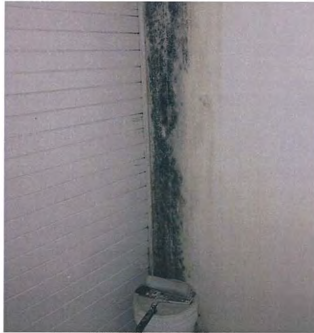
Photo11. Mold inside main house at first floor.
