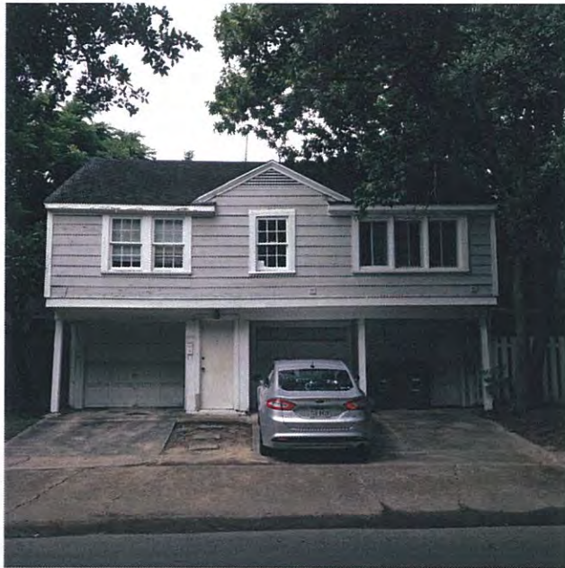
Photo15. Exterior elevation of garage apartment on Hazard Street. Sagging roof and floor cantilever.
