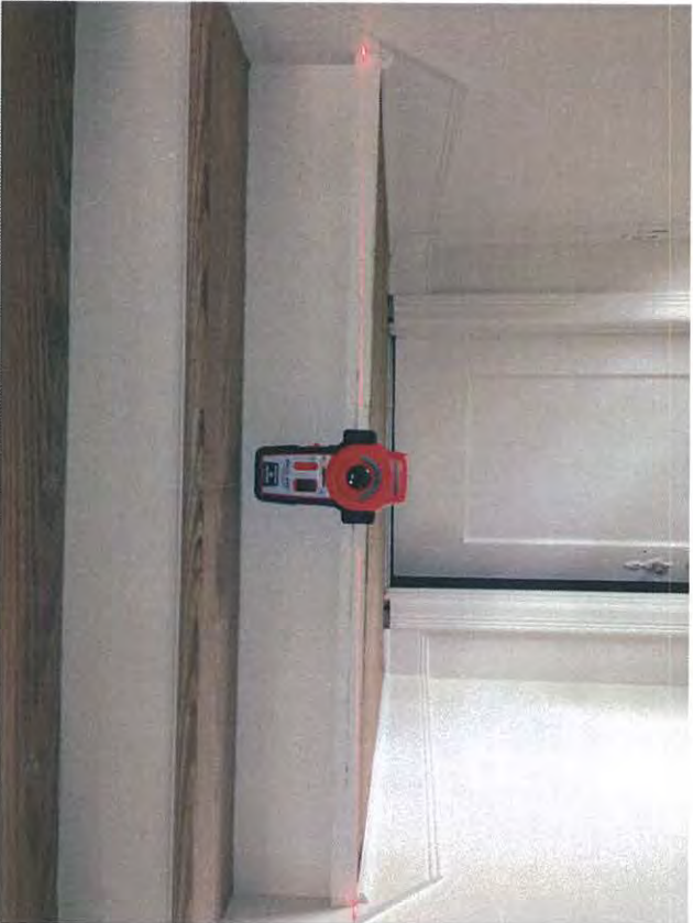
Photo6. Unleveled stairs at main house. Measured 1 inch drop along stair width.
