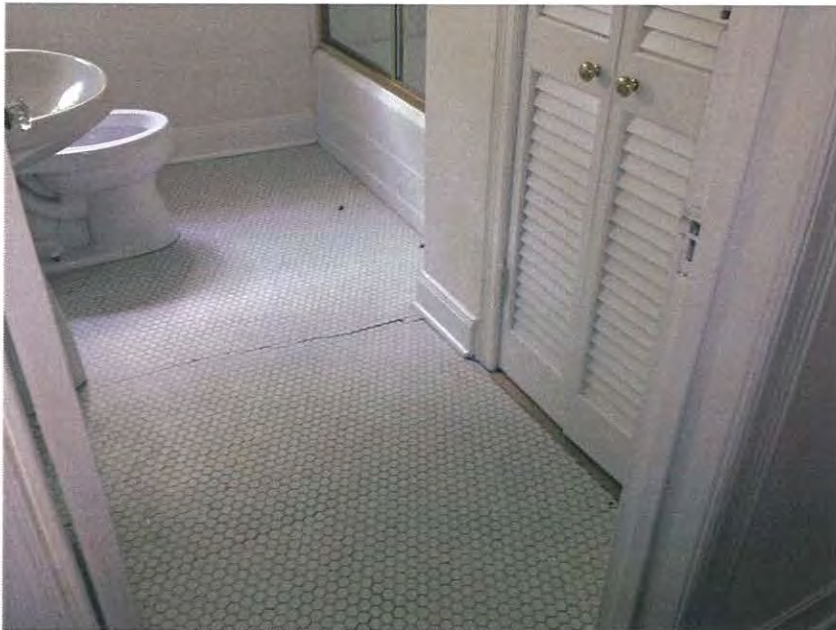
Photo8. Second floor bathroom at main house. Floor is cracked and unlevel. 2 inches drop from exterior wall to entrance door.
