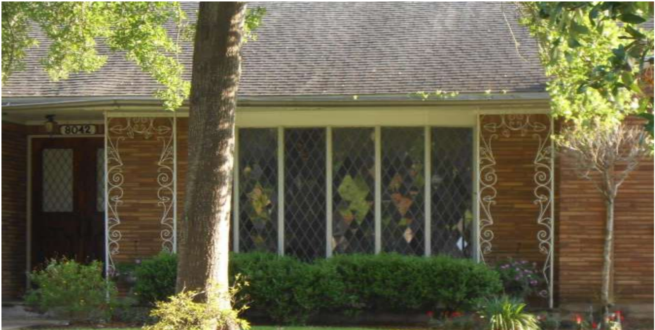
BAY WINDOW WITH ORIGINAL ALUMINUM WINDOWS AND NON-ORIGINAL FRONT ENTRY DOOR
