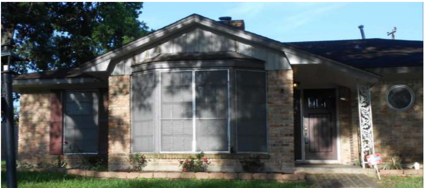
BAY WINDOW WITH ORIGINAL ALUMINUM WINDOWS AND NON-ORIGINAL FRONT ENTRY DOOR
