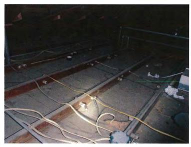
24. There was no insulation observed in the attic space. This is a source for significant energy loss.
