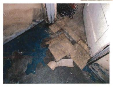
12. Interior floor coverings were tile. It was not determined if the floor tiles were asbestos type, and further testing is recommended.
