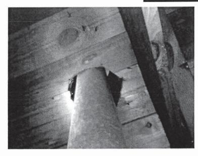
The double-wall pipe of the hot water heater for Unit 605 vent was touching combustible material. Double-wall pipes should have a clearance of 1inch minimum between any combustible surface and the wall of the pipe.
