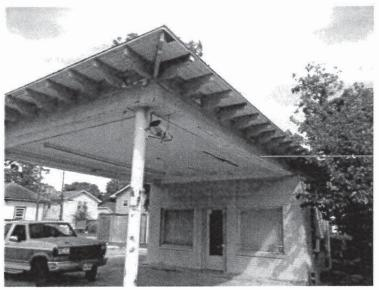
9. Abnormal sags could be observed in the roof joists of the carport cover and at the supporting beams. This is believed to be related to deterioration caused by water penetration from the roof, as some wood rot could be observed at the ceiling joists through the exposed open ceiling.
