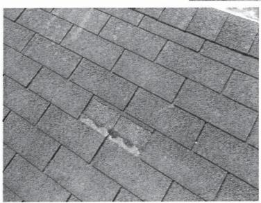
9. Shingle tabs were broken off at some locations, including at the east roof, leaving exposed nails and joints in the shingles that can allow water entry.
