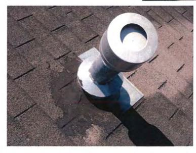
3. Roofing compound had been applied to the roof surface at the gas flue roof jacks, which would indicate a problem with water penetration. Roof compound is a temporary repair material and should not be necessary on a properly constructed roof. PHOTOGRAPHS – HOUSE STRUCTURE MARTINEZ
