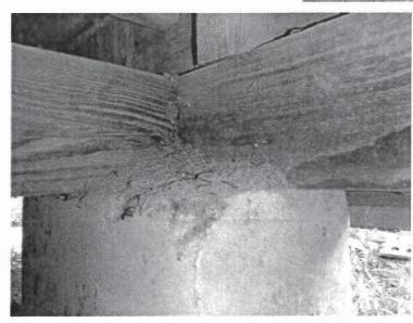
12. It is possible that minor wooddestroying insect damage to the structure exists at the north crawlspace below the living room of Unit 607 which could not be evaluated based upon a cursory inspection.
