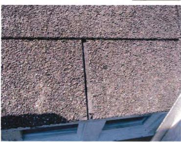
6. The starter strip shingles were installed upside down and were deteriorating at the first course shingle tab slots. As the starter strip erodes through, it will allow water penetration to the roof decking. PHOTOGRAPHS – HOUSE STRUCTURE MARTINEZ
