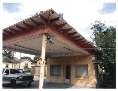
9. Abnormal sags could be observed in the roof joists of the carport cover and at the supporting beams. This is believed to be related to deterioration caused by water penetration from the roof, as some wood rot could be observed at the ceiling joists through the exposed open ceiling. PHOTOGRAPHS – GAS BUILDING STRUCTURE MARTINEZ
