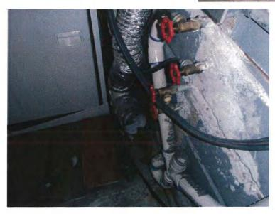
3. The dryer vent at the utility porch had an opening for an adjacent dryer that was not installed and was open to the porch. PHOTOGRAPHS – HOUSE MECHANICAL MARTINEZ
