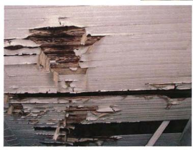
6. Paint was spalling off the ceiling, and the ceiling was rotting with missing planks at the main room due to water penetration from the roof above. Water penetration through the roof can rot the structure.
