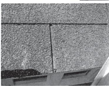
6. The starter strip shingles were installed upside down and were deteriorating at the first course shingle tab slots. As the starter strip erodes through, it will allow water penetration to the roof decking.
