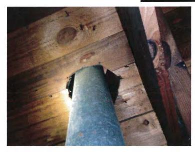
6. The double-wall pipe of the hot water heater for Unit 605 vent was touching combustible material. Double-wall pipes should have a clearance of 1inch minimum between any combustible surface and the wall of the pipe. **PROFESSIONAL ENGINEERING INSPECTIONS, INC.**
