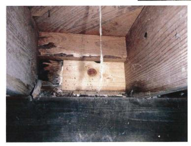
15. Siding was rotting behind the porches and can allow water to run past the siding and reach the girder beam, which may result in premature deterioration if the siding goes unprotected.
