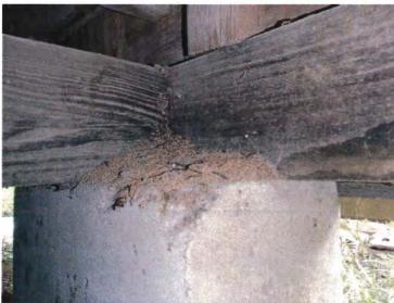
12. It is possible that minor wooddestroying insect damage to the structure exists at the north crawlspace below the living room of Unit 607 which could not be evaluated based upon a cursory inspection. PHOTOGRAPHS – HOUSE STRUCTURE MARTINEZ
